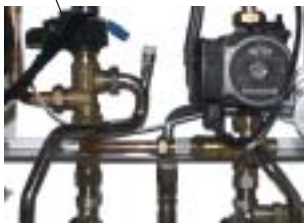
Three-way diverter valve
