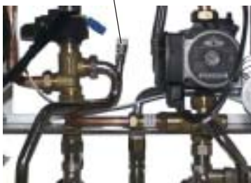
Vent - cylinder flow
