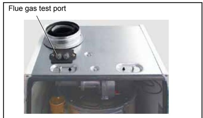
Fig.: Flue gas test with an open boiler
