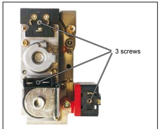
Fig.: Gas combination valve.
