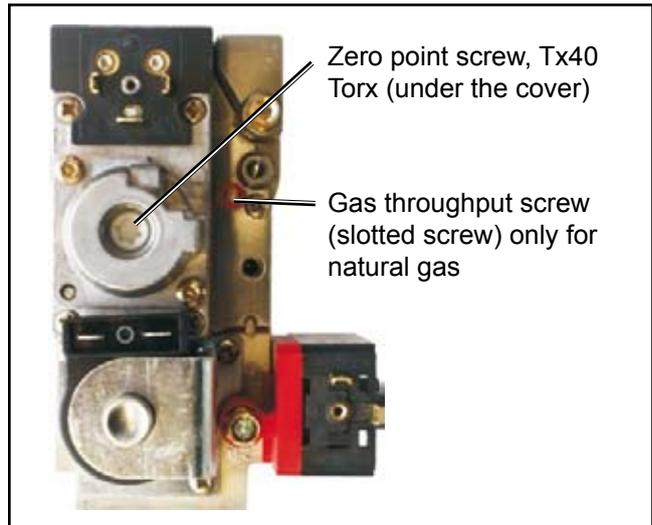
Fig.: Gas combination valve.
