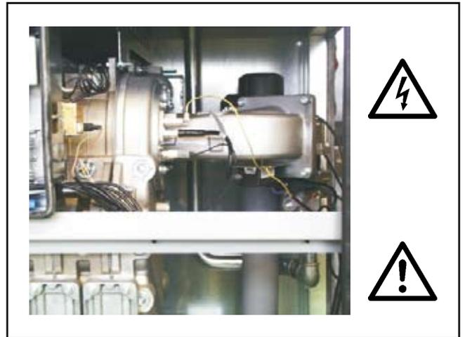
Fig.: Ignition transformer, high voltage ignition electrode, combustion chamber.
