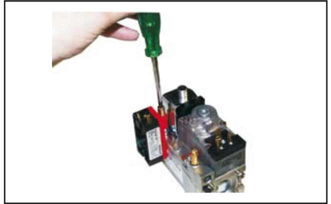
Undo and remove the screw for the gas supply pressure on the new gas combination valve.
