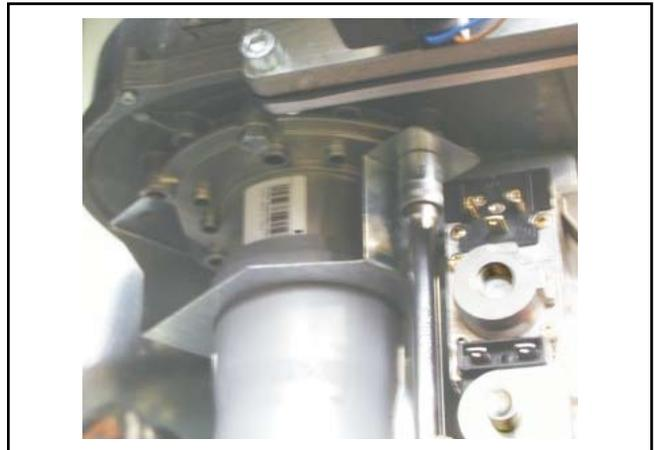
j) Secure the electrical connections on the GCV.
